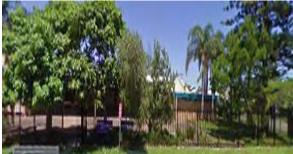
Pelican Flat Public School - Formerly Marks Point School until Sep 1950 (Google Street View 2010)
