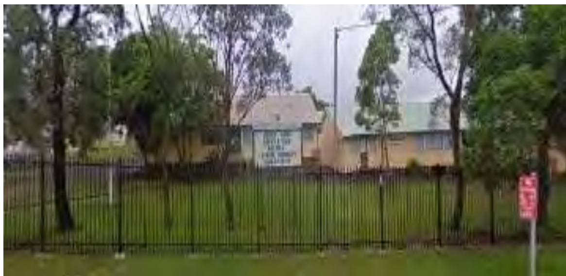
Argenton Public School (Google Street View – 2010)
